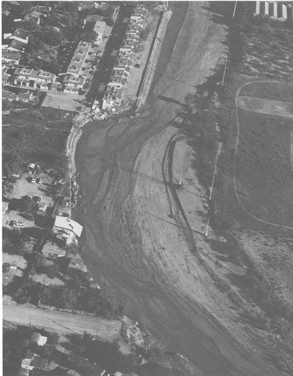
FIGURE 6. Damage to the Pima Park Townhomes caused by lateral migration of a prominent meander bend of Rillito Creek. Erosion occurred behind the soil cement bank protection shown adjacent to the townhomes, leading to its failure. Photograph by Peter Kresan.
