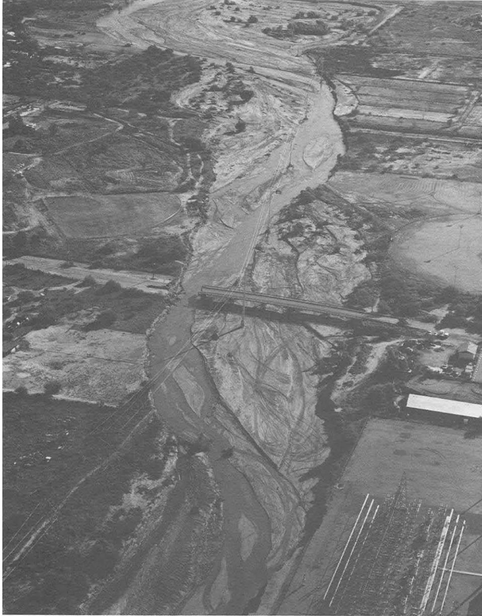
FIGURE 5. Damage to the northern (left) abutment of the Dodge Road bridge across Rillito Creek caused by channel bank erosion and lateral channel migration in October, 1983. Note the threat to the electric utility station on the opposite bank downstream. Photograph by Peter Kresan.
